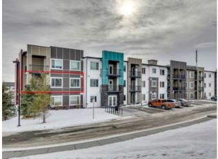
Cement Fiber Board, Composite Siding
